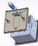
Screw the thermostat back plate on to the back box
