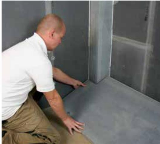
**2** Lay the Marmox Multiboard down onto the adhesive and push firmly.
