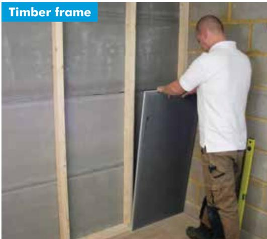
**1** For a stud wall built at 600 centres use 20mm Marmox Multiboard or thicker. 400 centres use 12.5mm and 300 centres use 10mm. Thinner than 10mm should not be used on stud walls.
