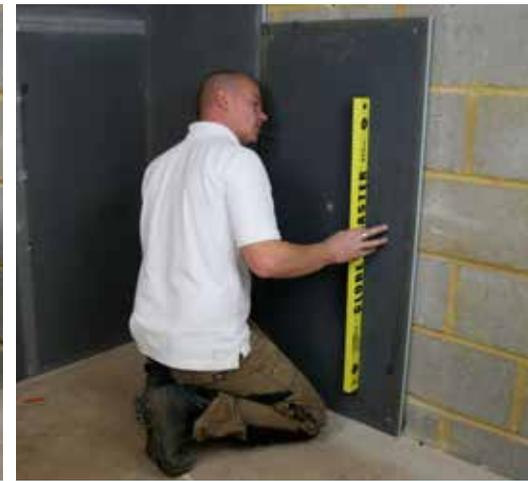
**3** Offer the Marmox Multiboard up to the wall, push firmly and then level with spirit level.
