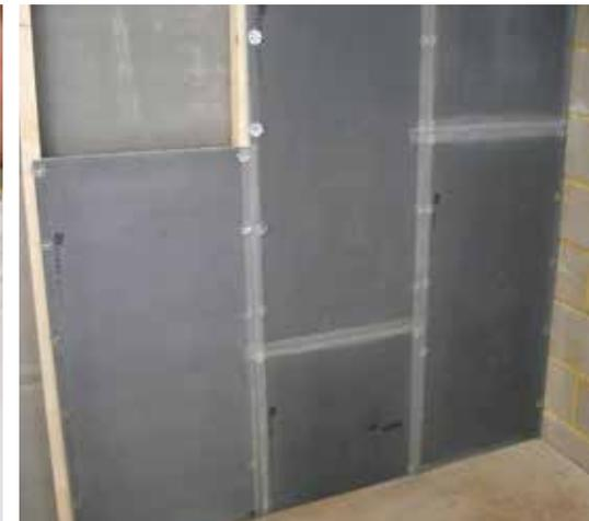
**3b - Plastering.** Seal boards together using a bead of Multibond prior to scrim-taping, do not use Waterproof tape under plaster. The boards are now ready to be plastered.
