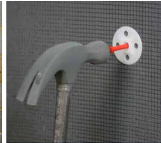
**4** Once the adhesive has dried drill the holes out. Place the white dowel in through into the wall and then hammer in the pin.
