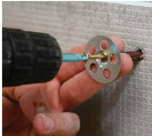
**2** Marmox Multiboards can be fixed to solid wall with screws and washers at every 300mm. Alternatively use Marmox Fixing Dowels for ease.
