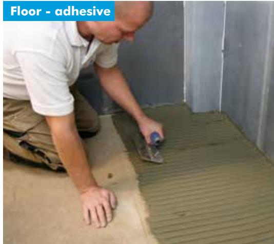
**1** Use a floor trowel to comb the adhesive onto the floor.
