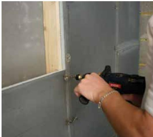
**2** Use a screw/Marmox washer at every 300mm. When timber is at 600 centres use 2 rows of 5 fixings. At 300 centres use 3 rows of 4 fixings.
